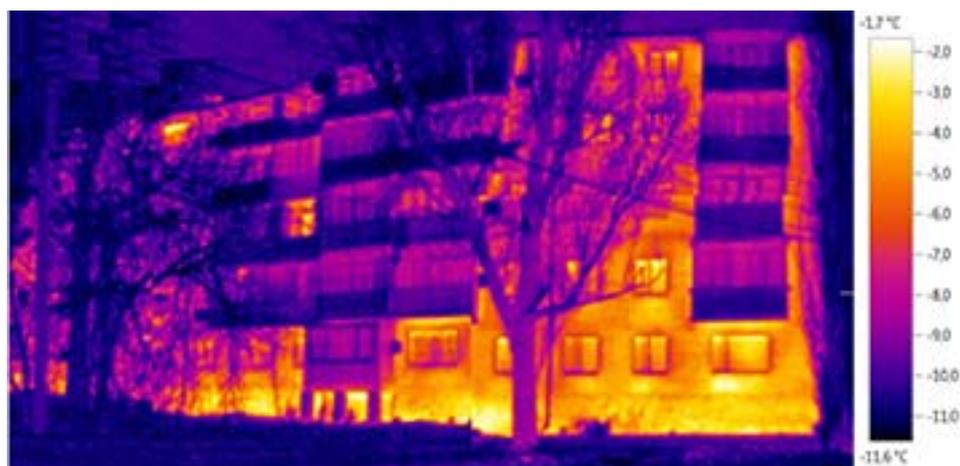
The natural research study let the authors point out the basic ideas that the front parts of the house, and bricklaying parts have some abnormal zones (i.e. the zones with increased temperature appeared on external surface of protecting designs at the expense of ex filtration).
